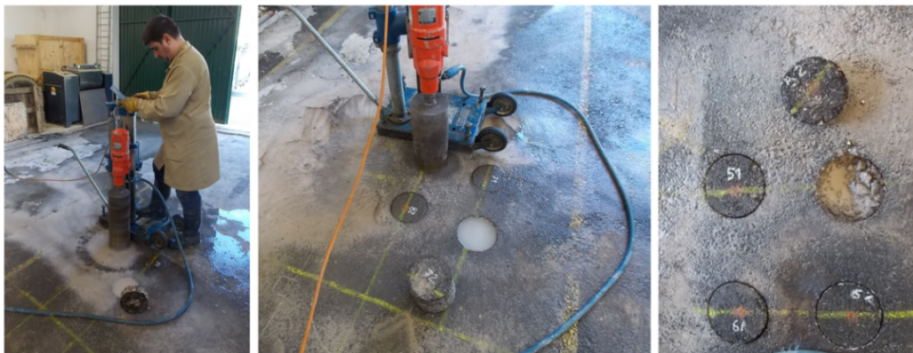
Fig. 6 – Extraction of drill cores.
