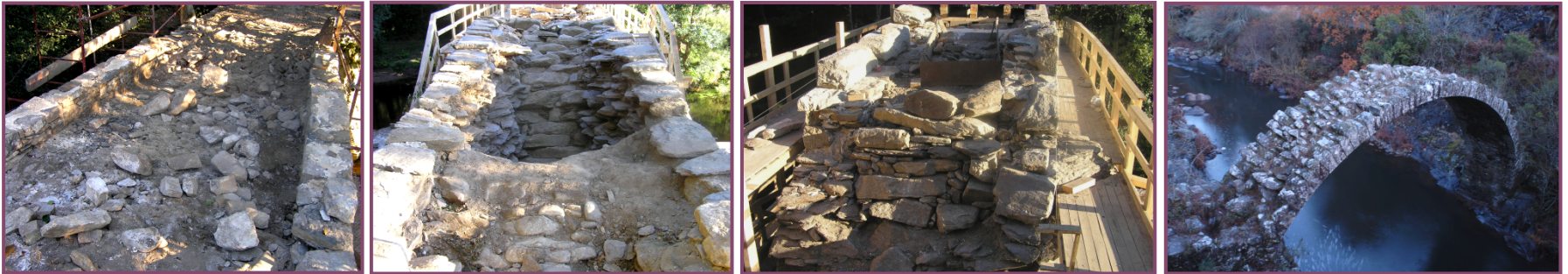
Fig. 1. Non-homogenous filling within the San Albert Bridge during the restoration tasks performed in 2006 and irregular shape of ring-stones in the Carixa Bridge.
