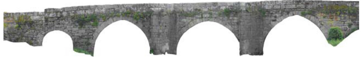
Fig. 6. Orthophoto of the upstream wall of the Traba Bridge produced by laser scanning methods.
